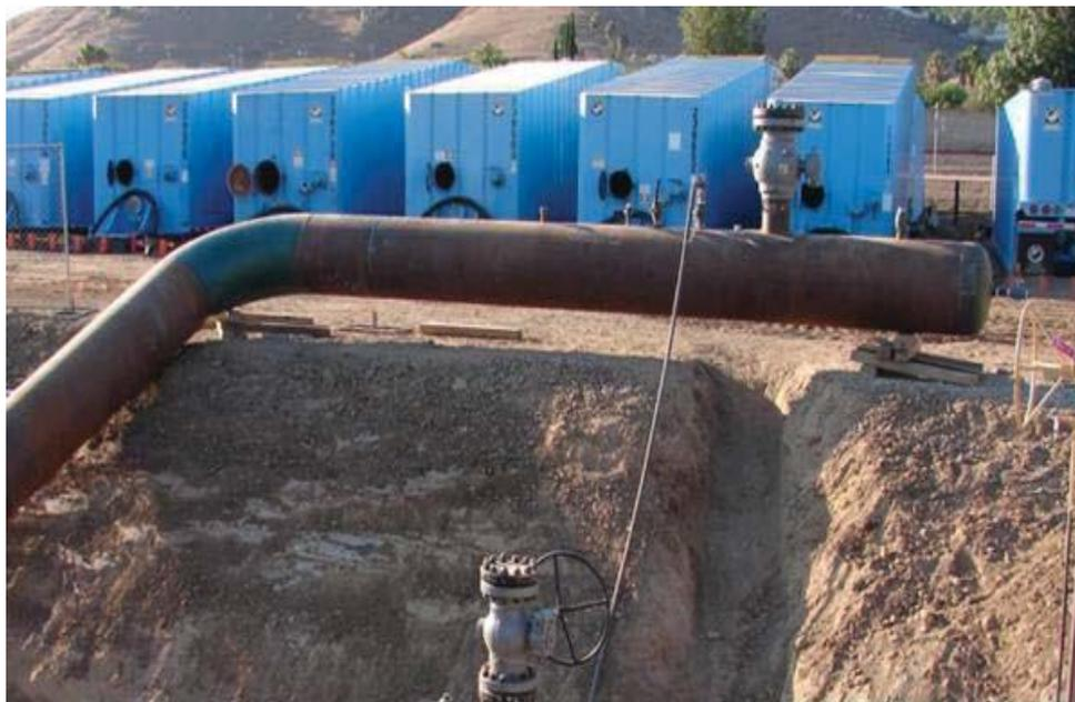
Figure 14: L-2000 Tie-In Construction
