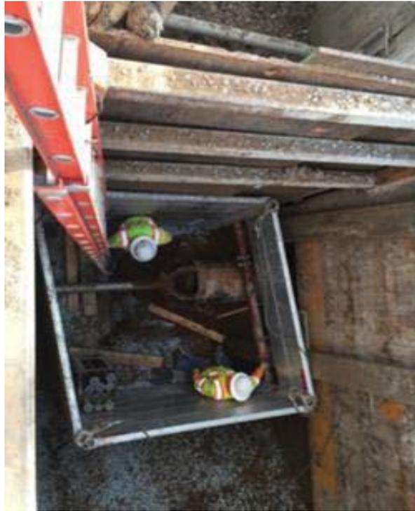
Figure 8: Jack and Bore Operation
