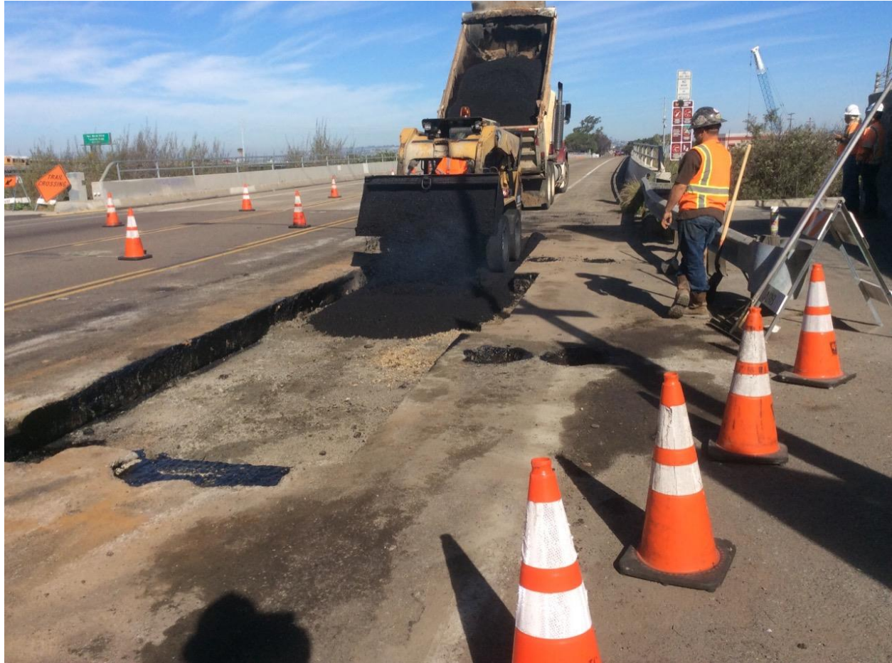
Figure 5: Bell Hole Paving
