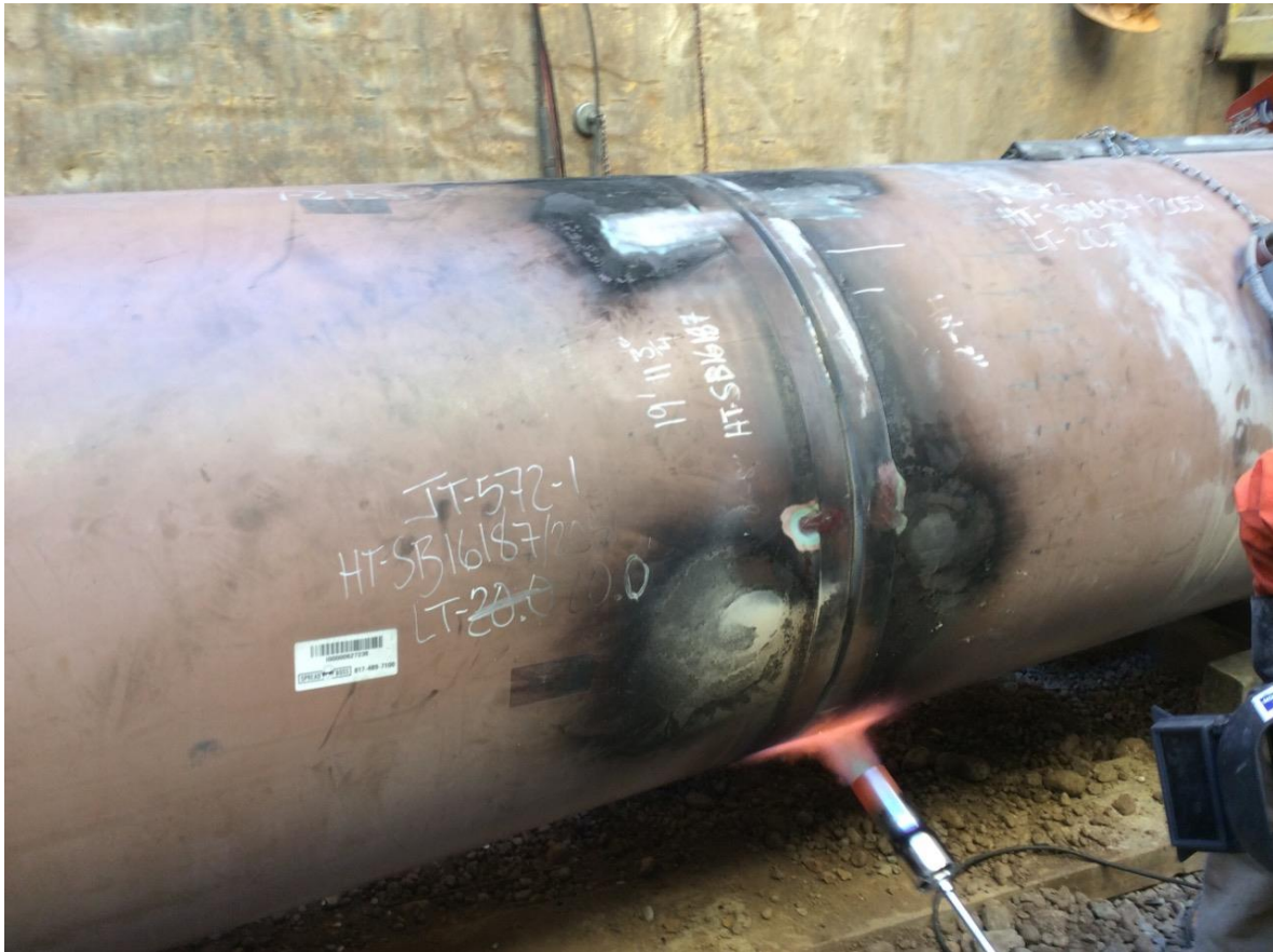
Figure 8: Preheating of Casing Pipe Between Welding Passes
