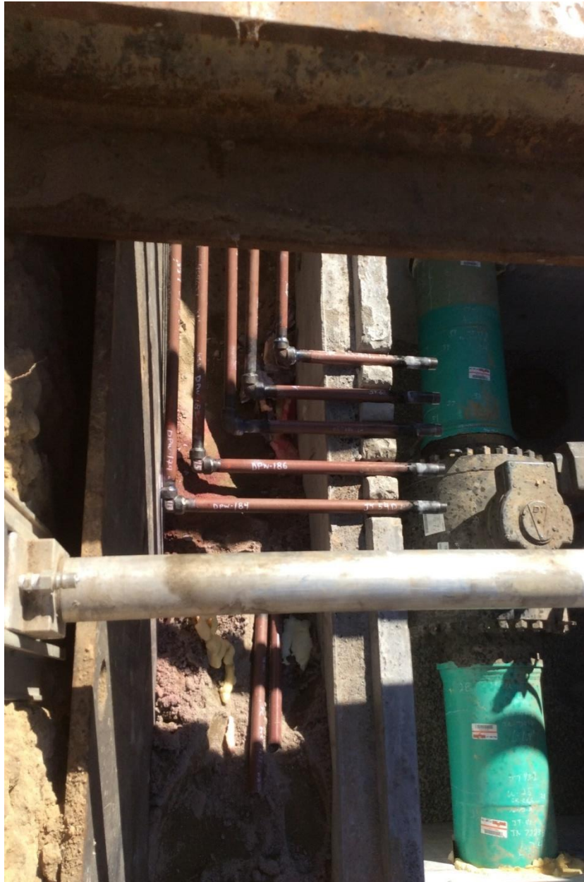
Figure 4: New Sensing Lines
