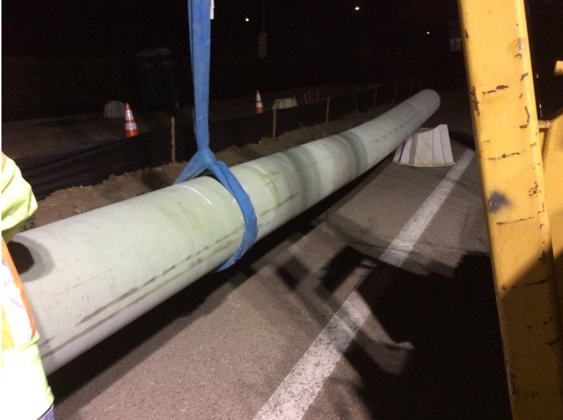
Figure 7: Pipe With Field Bend
