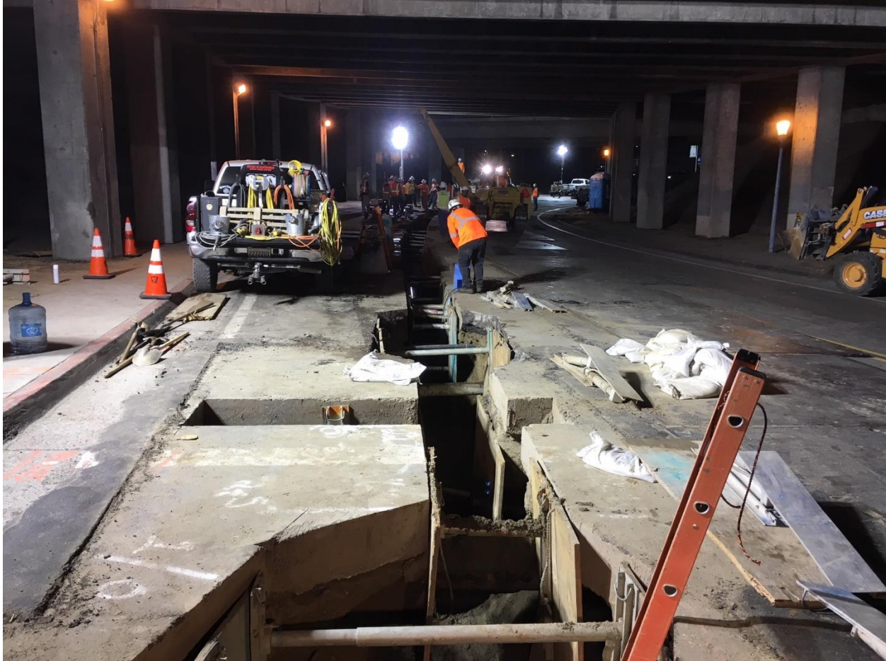
Figure 5: Nighttime Trenching Under the Interstate 8 Freeway
