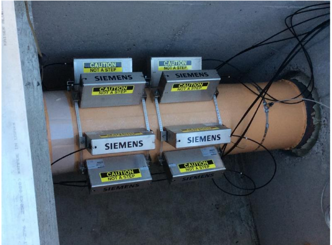
Figure 3: New Clamp On Flowmeter
