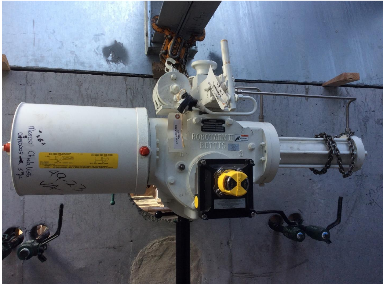
Figure 3: New Actuator in Vault during construction
