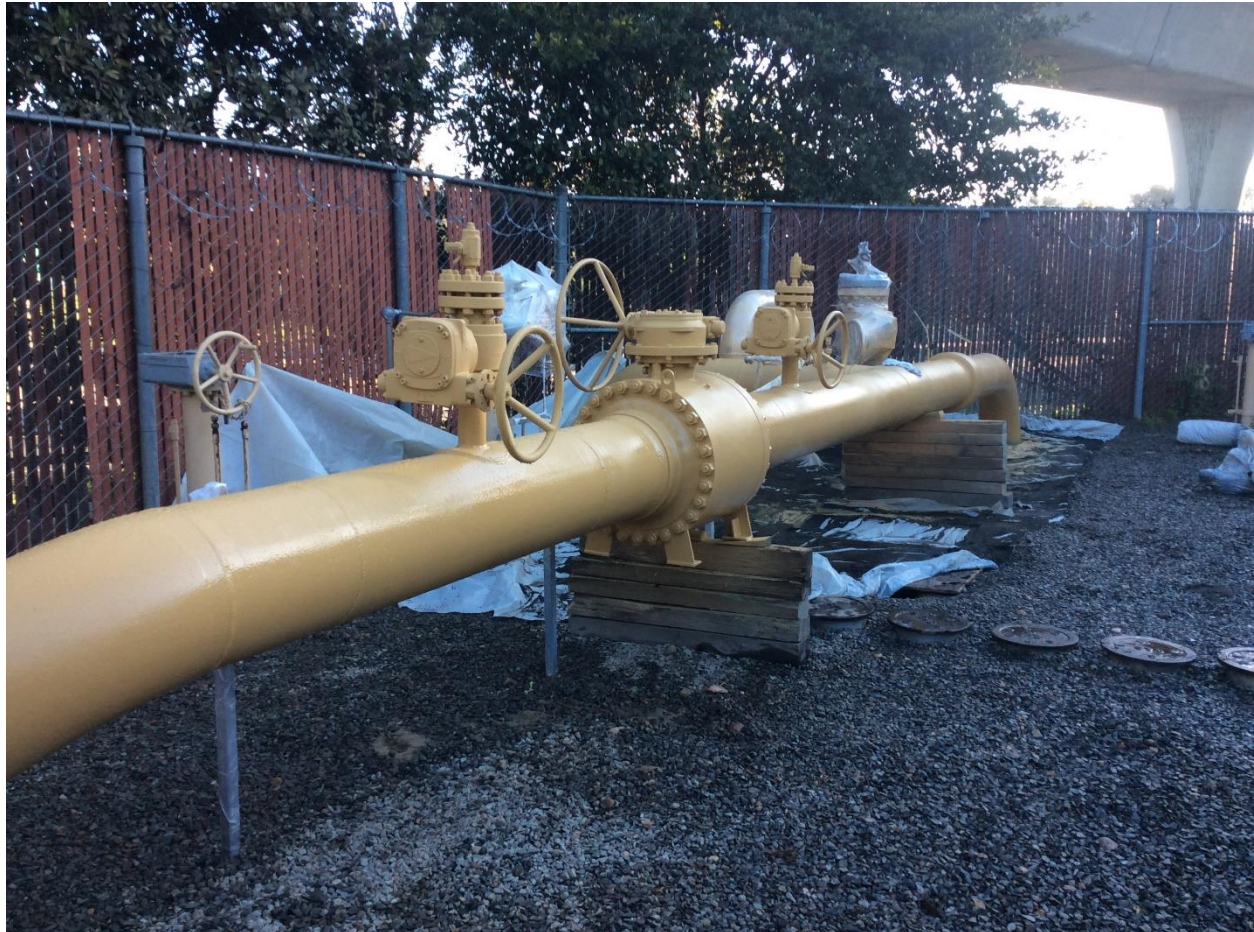
Figure 5: New Above Grade MLV
