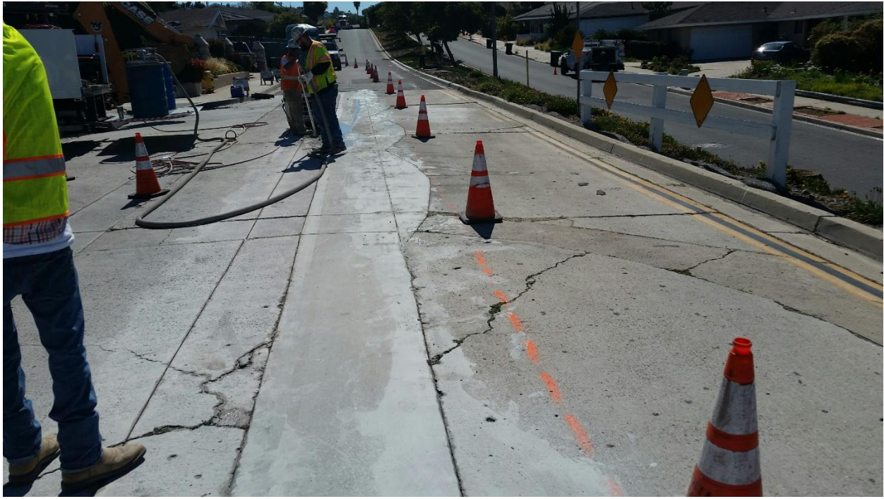
Figure 10: Saw Cutting Operations
