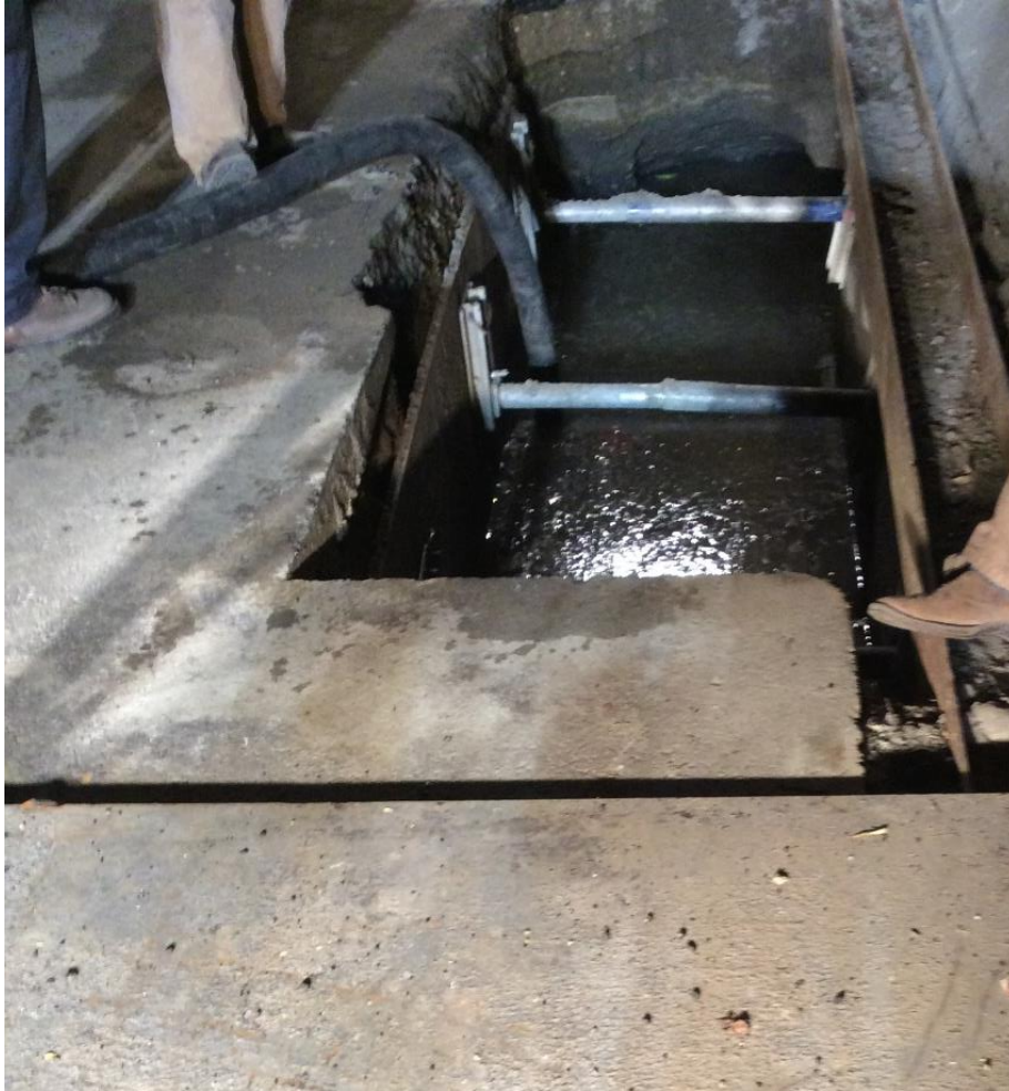
Figure 9: Groundwater Removal from Trench
