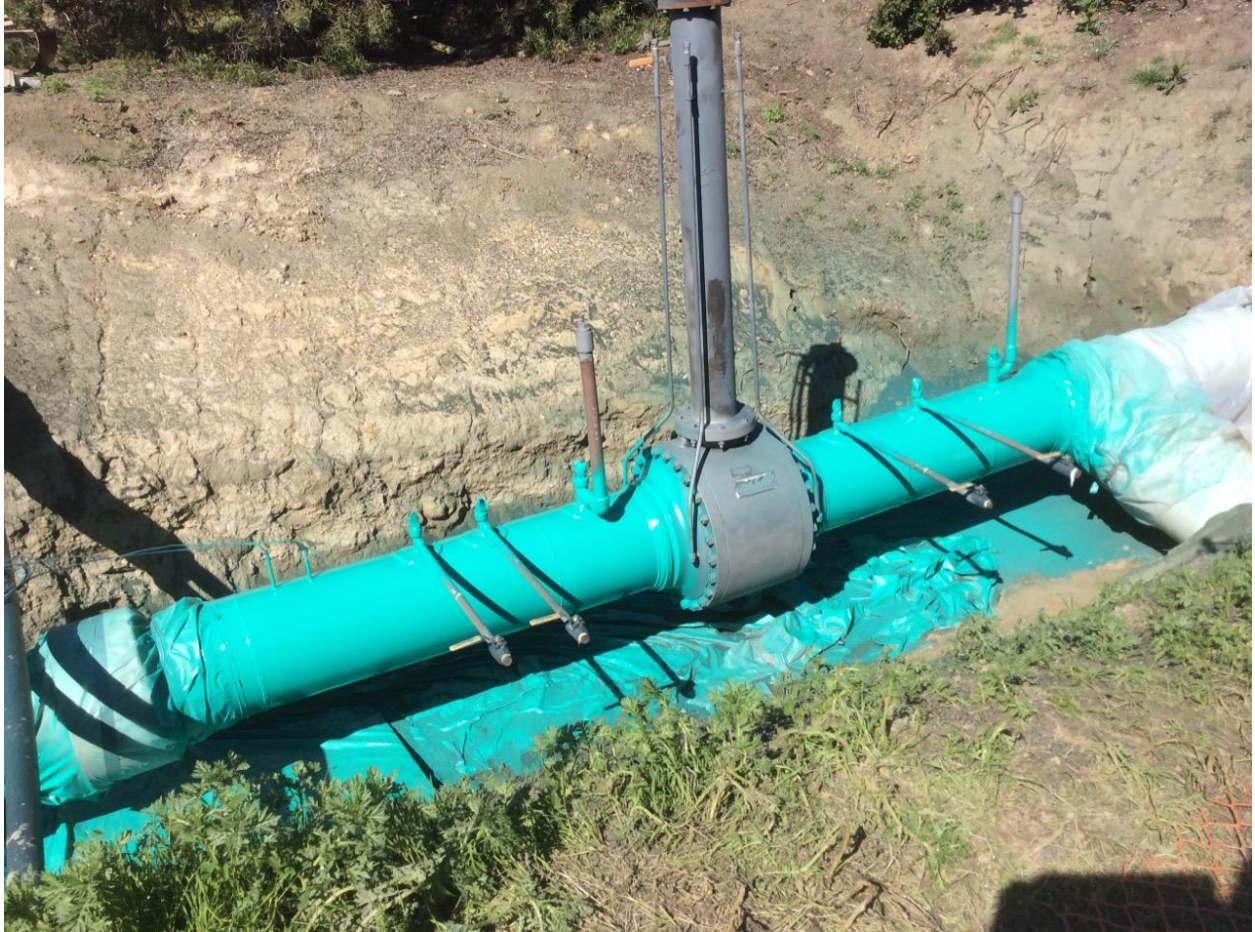
Figure 3: Mainline Valve Assembly With Instrument Piping
