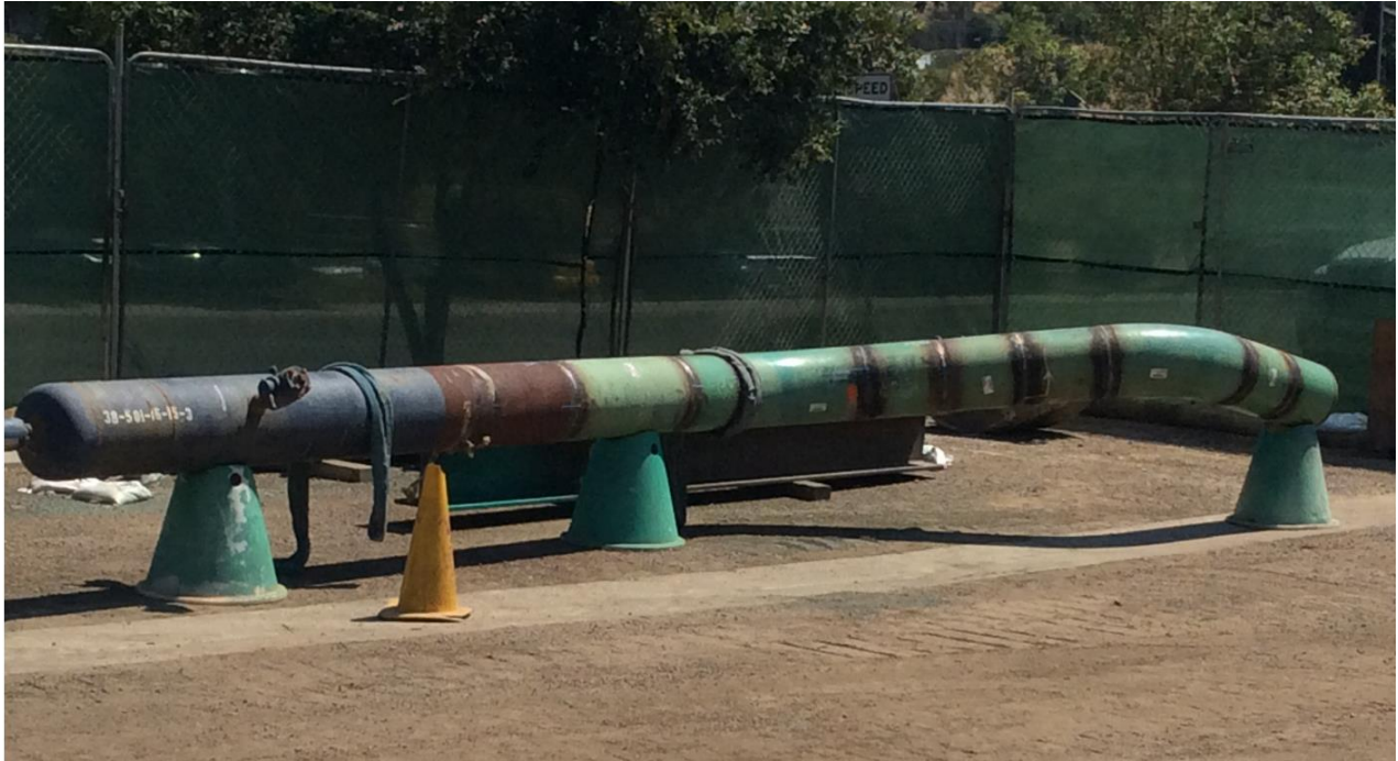
Figure 4: Section 4 Hydrotesting of a Prefabricated Installation
