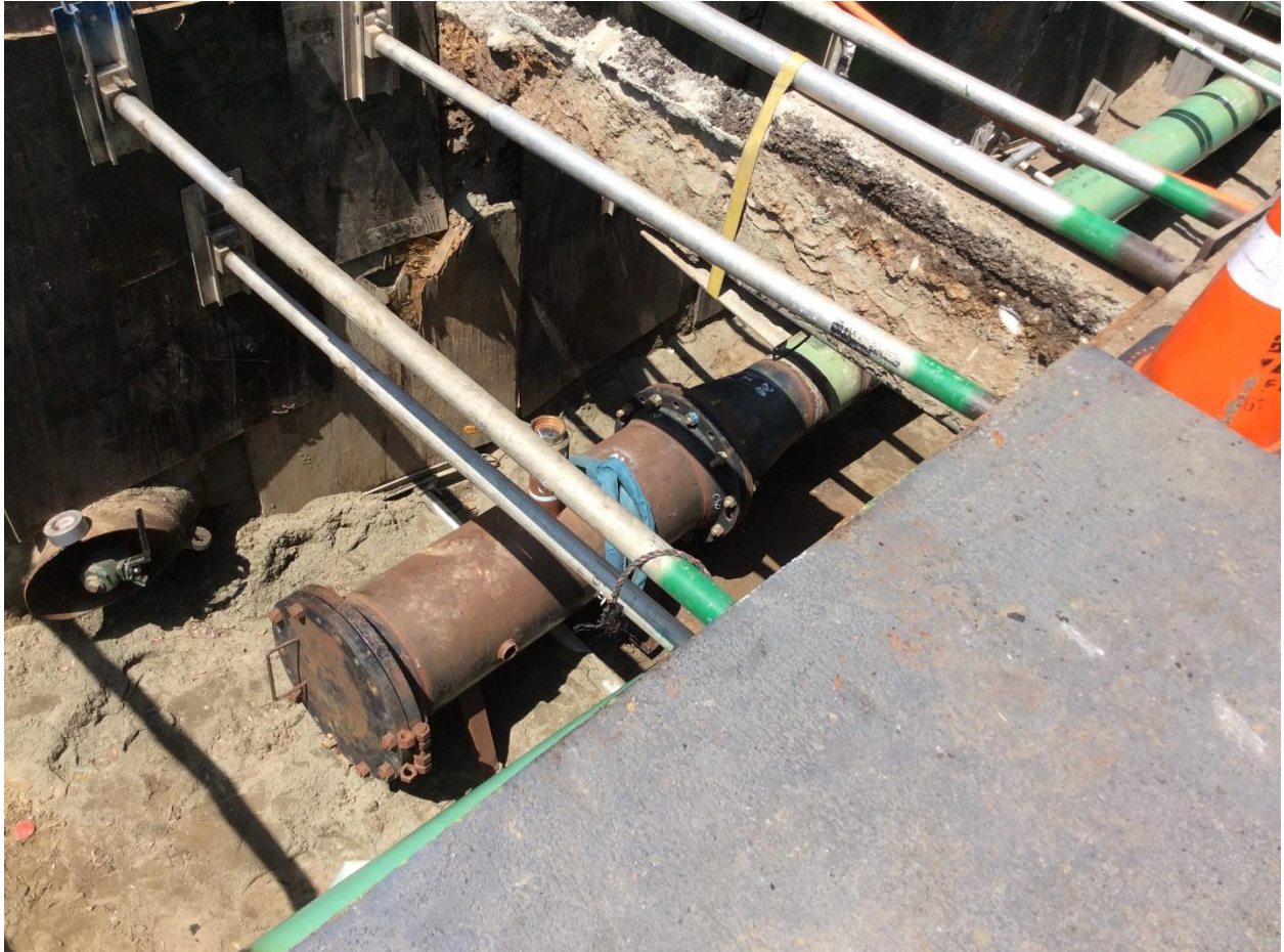
Figure 10: Pig Launcher for Post Completion Hydrotest
