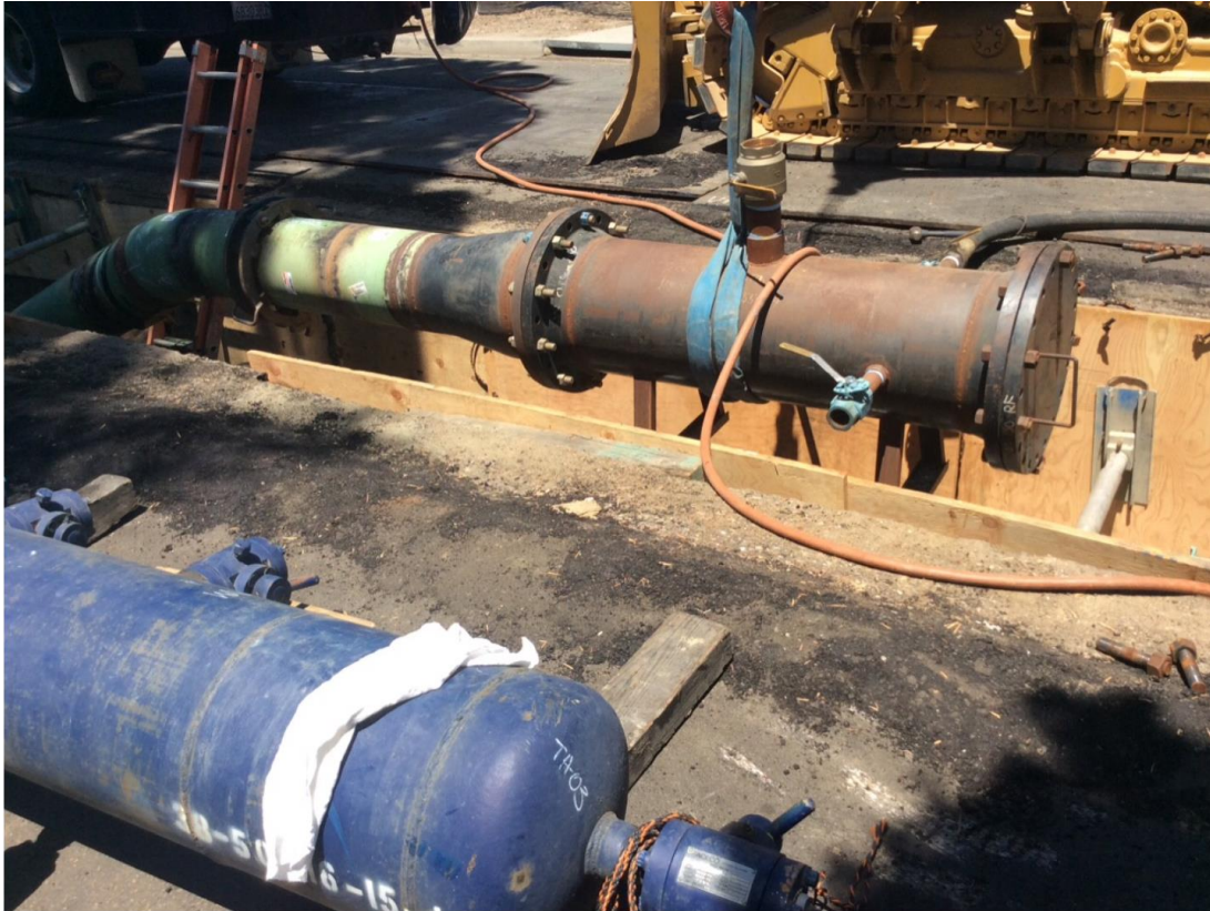
Figure 6: Section 6 Test Head in the Foreground, Temporary Pigging Equipment in the Background
