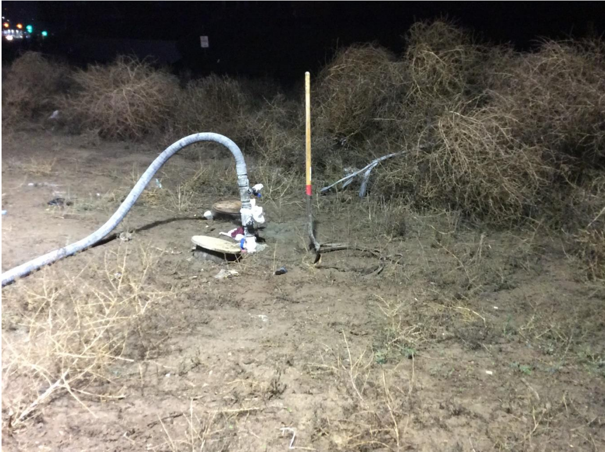
Figure 5: Grout Filling the Abandoned Pipeline
