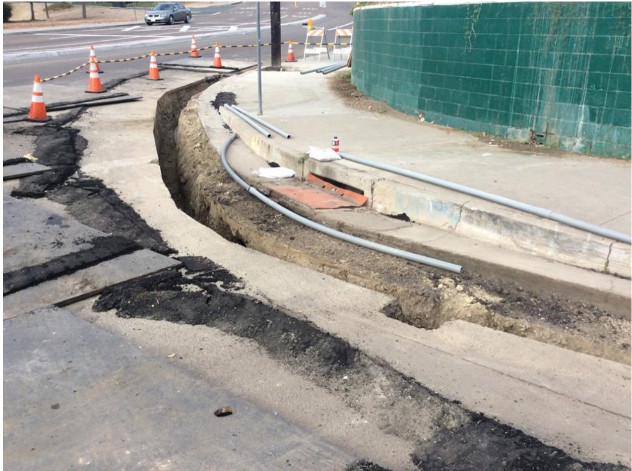
Figure 8: Trenching Work for Electrical Power Supply Installation at the Massachusetts and Main Site
